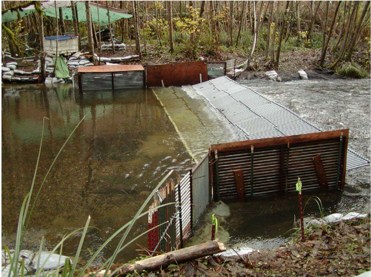
Photo 1. Resistance board weir Prairie Creek, Humboldt County, California during 2006/07 spawning season.
