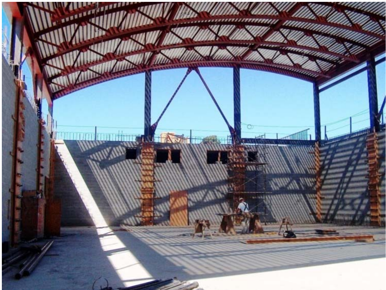
Wall construction in practice gym rises to the top.
