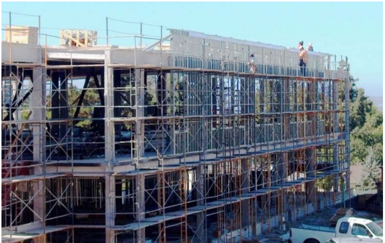
Exterior wall and parapet construction of Building B makes progress.
