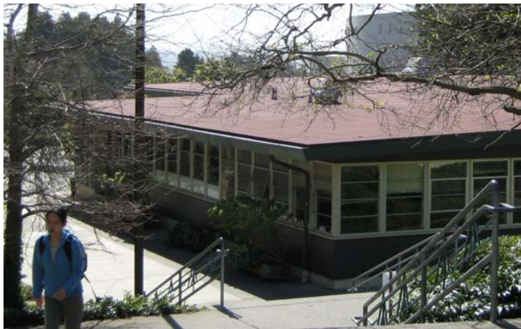
Figure 1: View of Old Music Building roof from main quad
