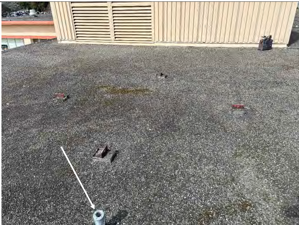
Photograph 10 – Humboldt Bay Aquatics Center – Exterior – Balcony – Vent flashing containing lead (typical)
