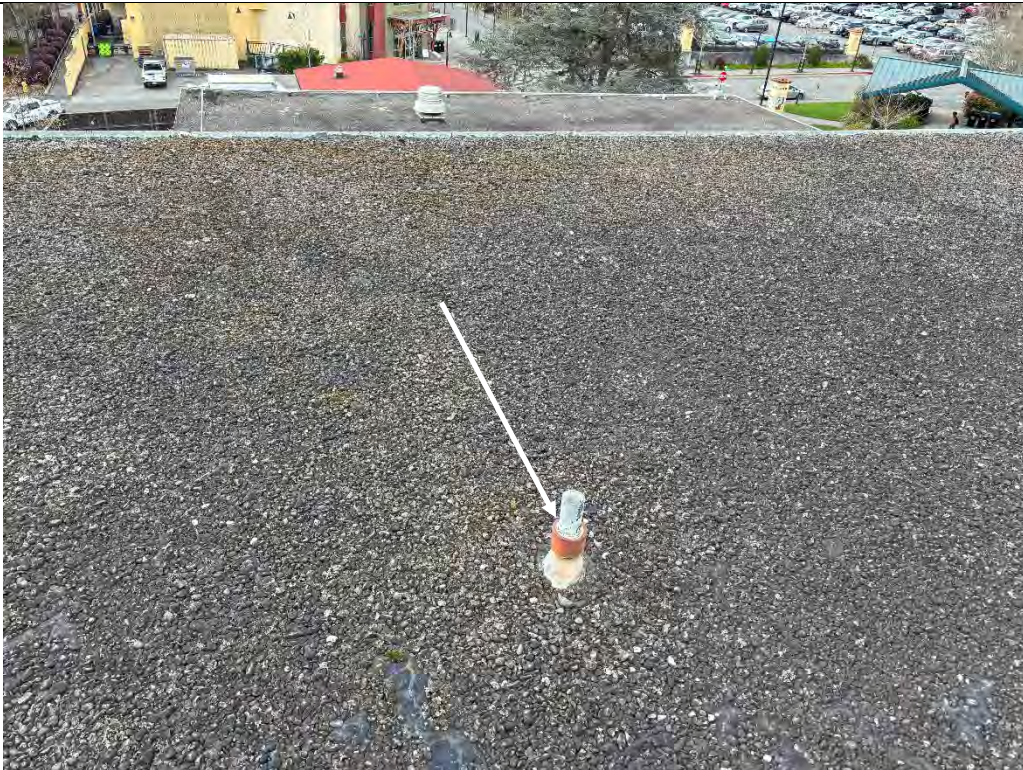
Photograph 8 – Exterior – Penthouse Balcony – Vent sealant reported to contain asbestos
