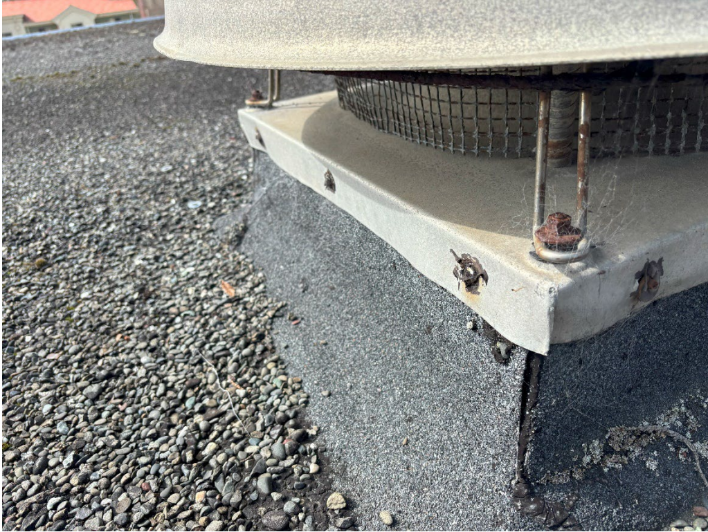
Photograph 9 – Harry Griffith Hall – Exterior – Roof – Vent flashing detail
