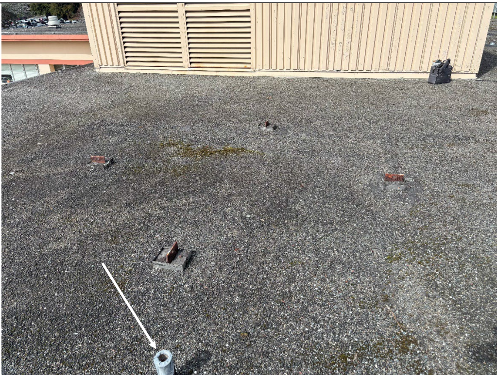
Photograph 10 – Harry Griffith Hall – Exterior – Roof – Vent pipe flashing containing lead (typical)
