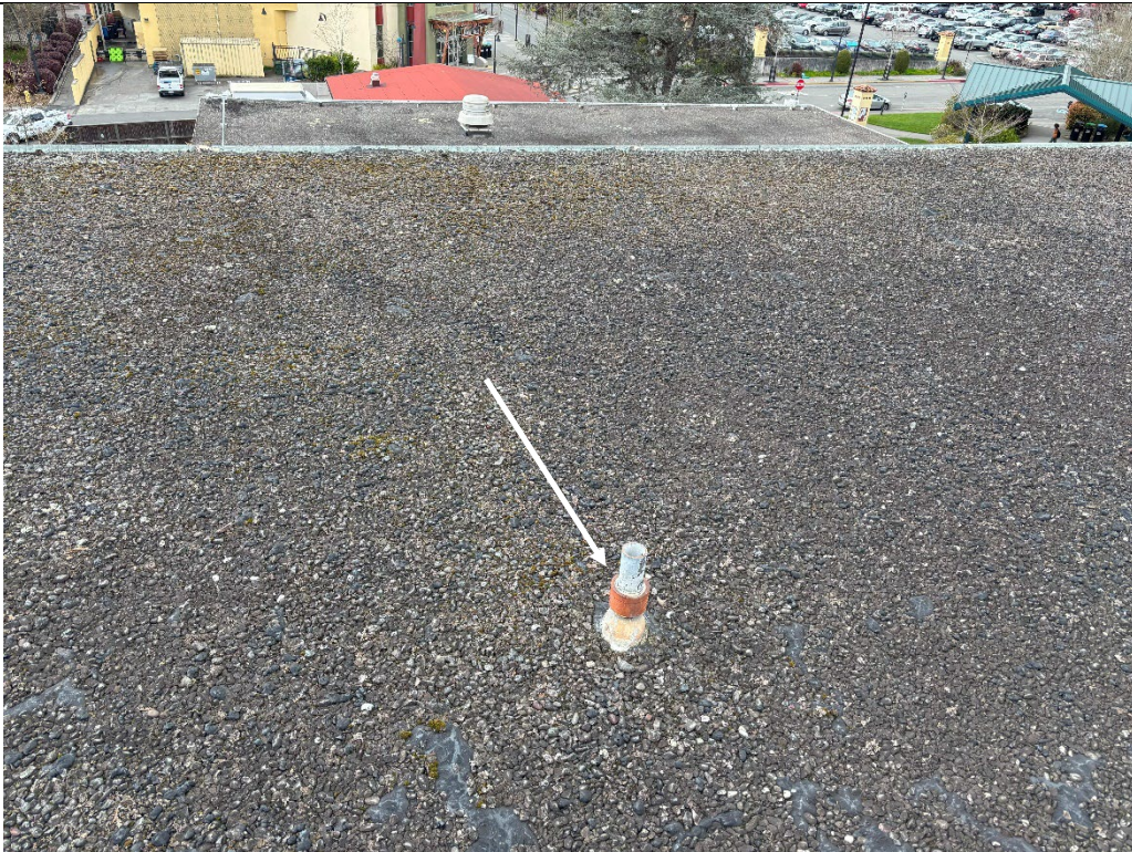
Photograph 8 – Exterior – Penthouse Roof – Vent sealant reported to contain asbestos
