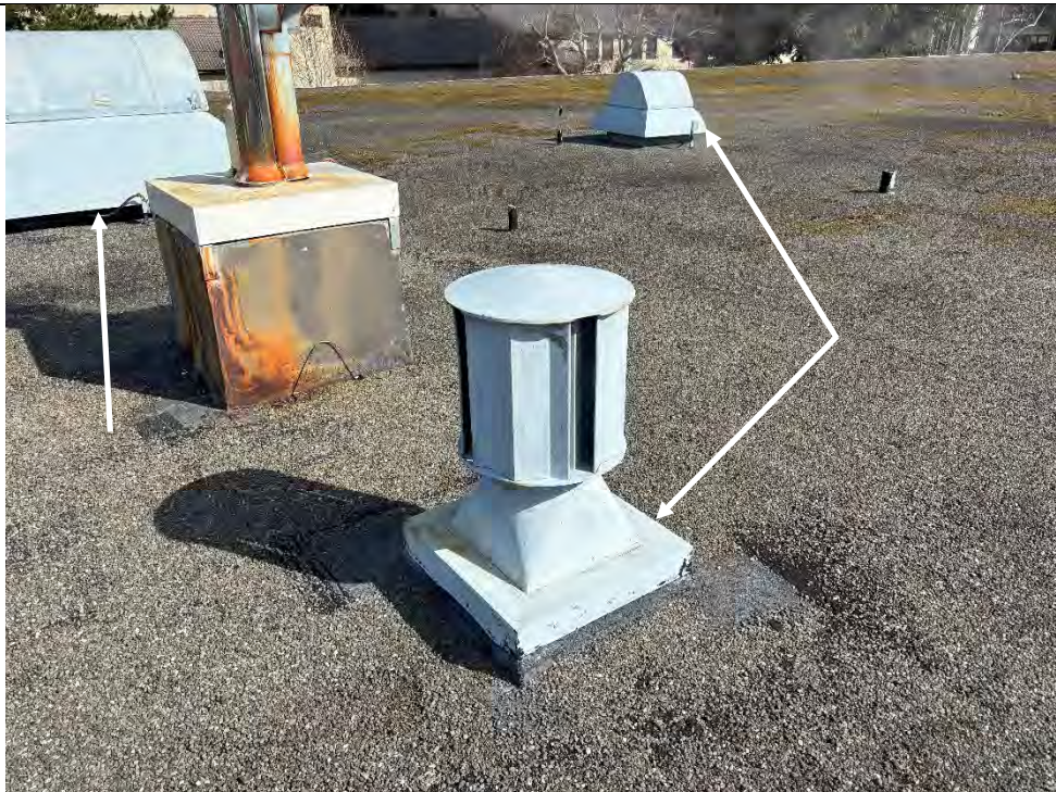
Photograph 8 – Exterior – Roof – HVAC vent housing paint (grey) containing lead (typical)
