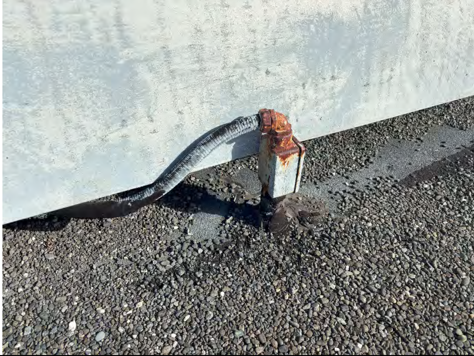
Photograph 5 – Siemens Hall – Exterior – Roof – Penetration mastic (black) (typical)
