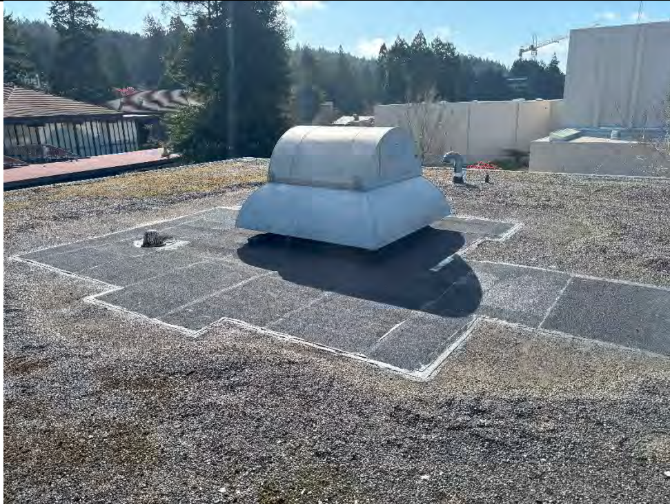
Photograph 7 – Siemens Hall – Exterior – Roof – Rolled roofing patch at southwest-center
