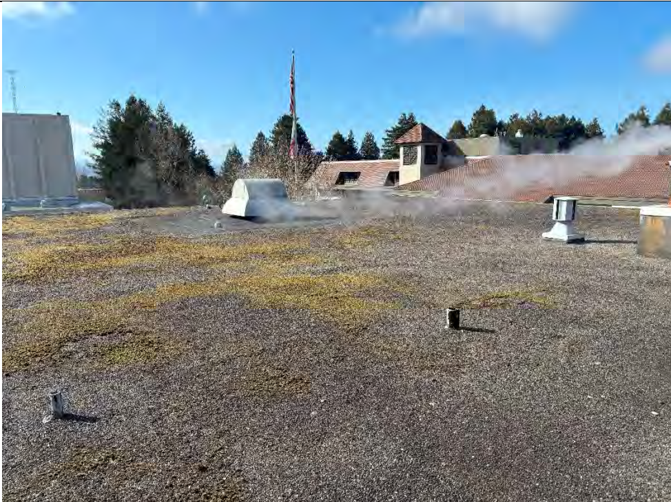
Photograph 4 – Siemens Hall – Exterior – Roof – View looking southwest – Built-up roofing (typical)
