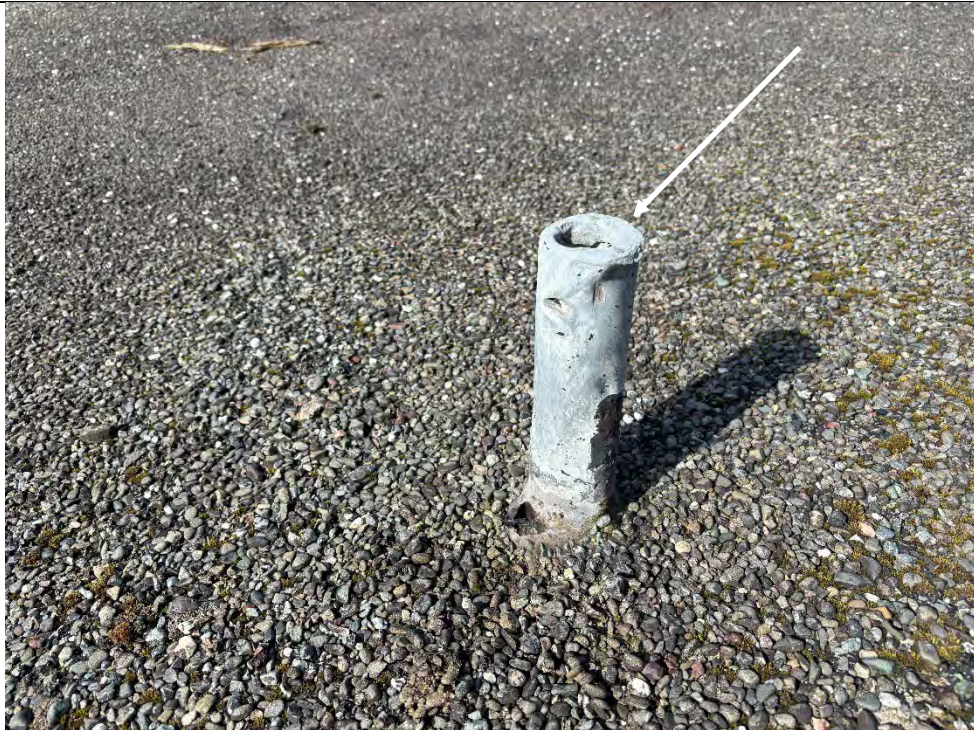
Photograph 6 – Siemens Hall – Exterior – Roof – Vent pipe flashing containing lead (typical)
