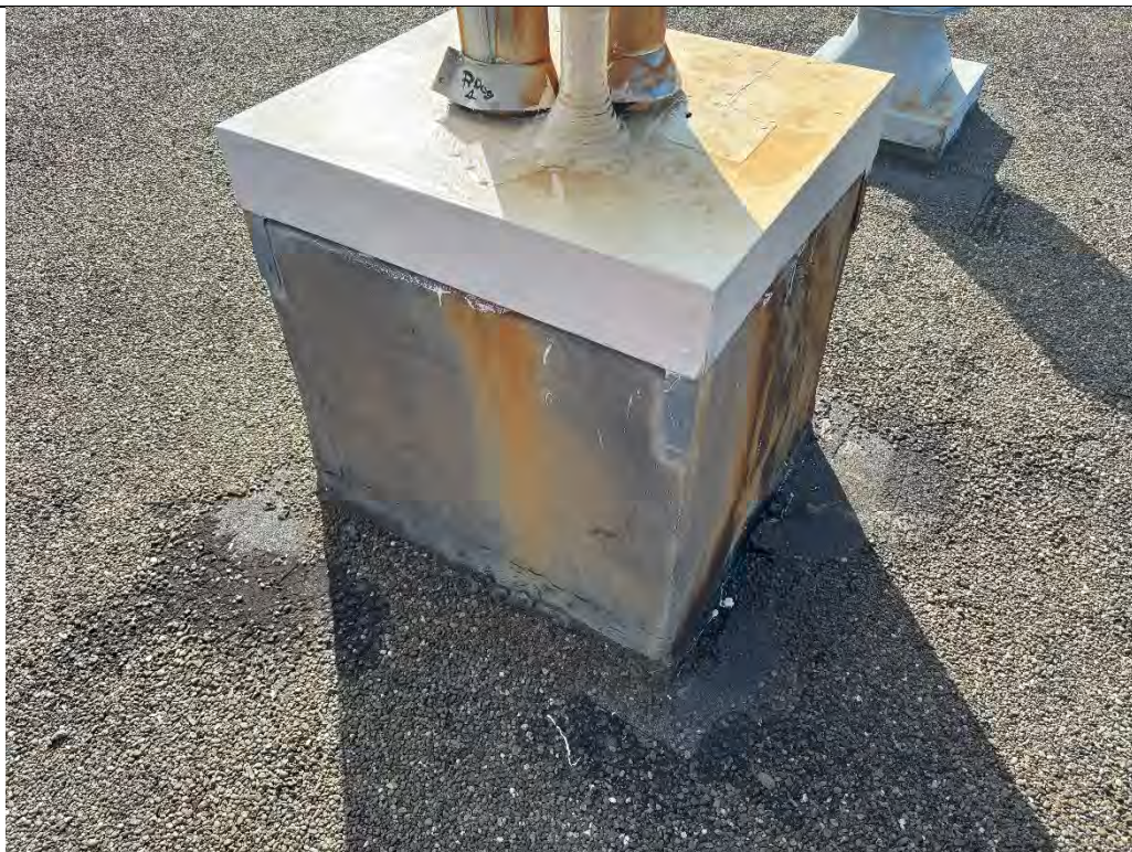
Photograph 10 – Siemens Hall – Exterior – Roof – Vent curb epoxy coating (black)
