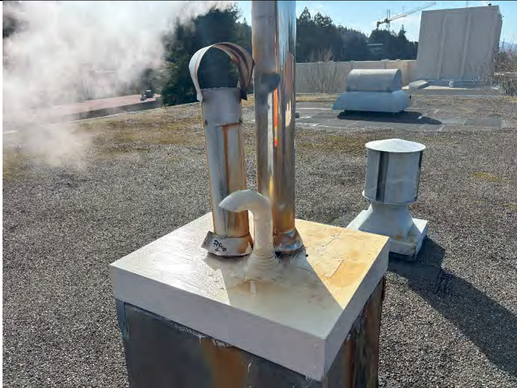
Photograph 9 – Siemens Hall – Exterior – Roof – Vent curb, flashing
