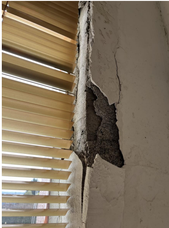
Figure 7 – Perimeter concrete wall at second floor with plaster finish.
