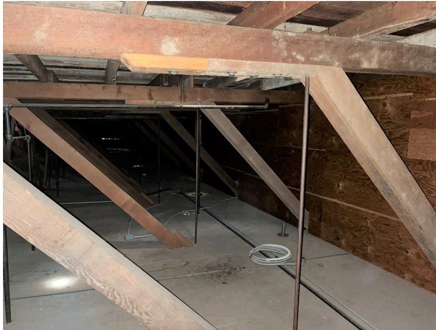
Figure 10 – Plywood walls and diaphragm below high roof
