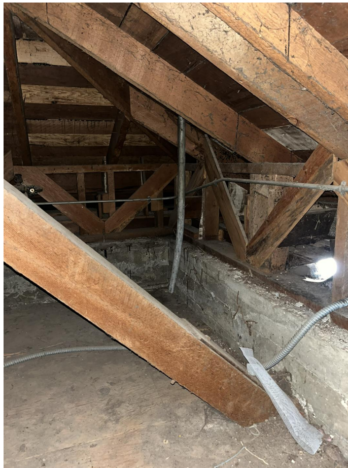
Figure 11 – Cripple wall with diagonal bracing on top of concrete wall at high roof
