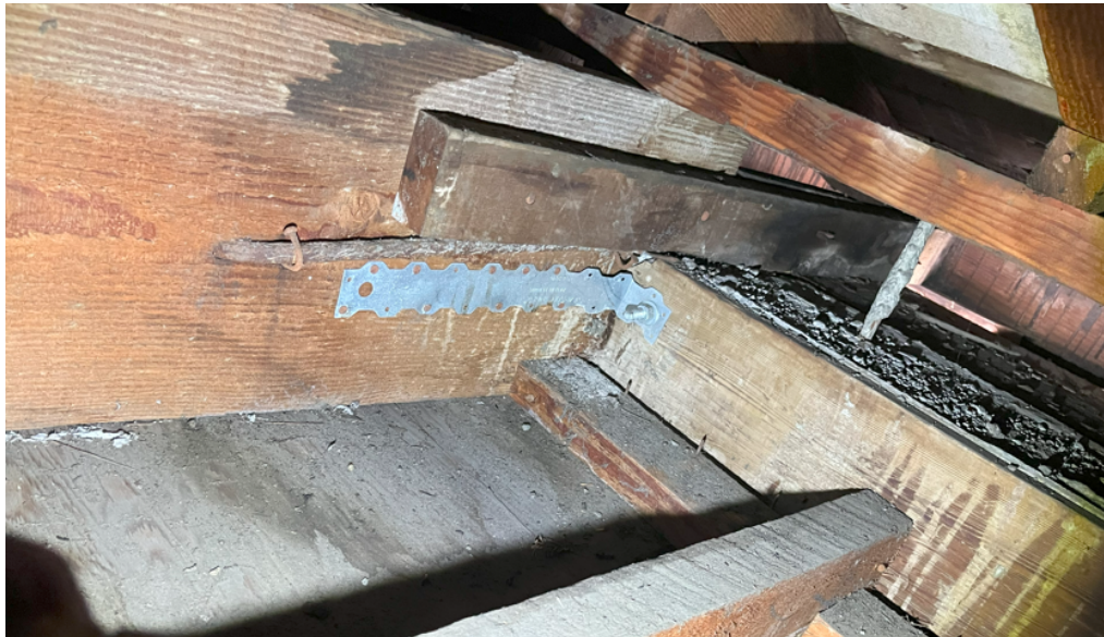
Figure 9 – Out-of-plane wall anchored to attic joist with plywood below.
