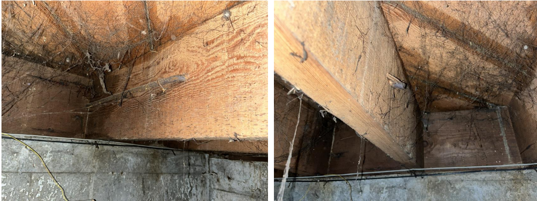
Figure 12 – Rebar extending out from the concrete wall and hooked through a second floor joist
