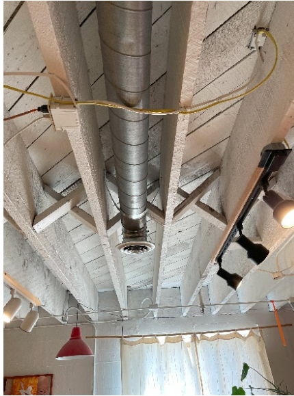
Figure 6. Level 1 Art Studio Duct and Diffuser
