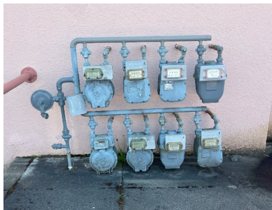
Above: Gas service and gas meters into building
