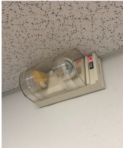
Figure 13. Emergency Lighting Unit
