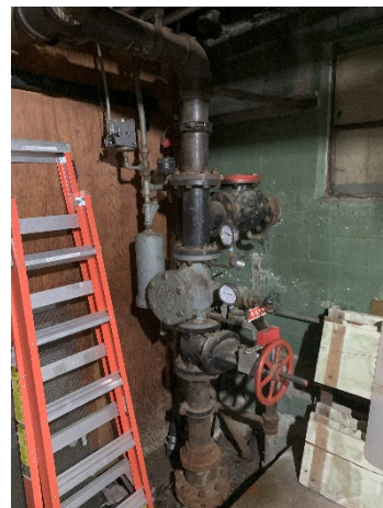
Above – Firewater Backflow Assembly
