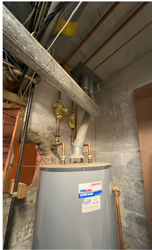
Above: Water heater with uninsulated domestic hot water piping
