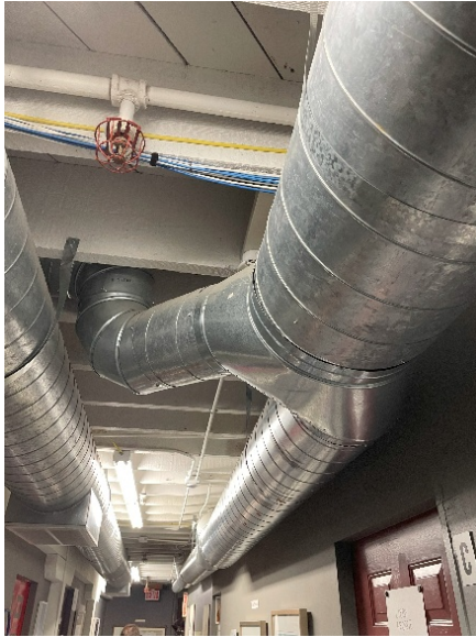
Figure 5. Level 1 Corridor Duct Main
