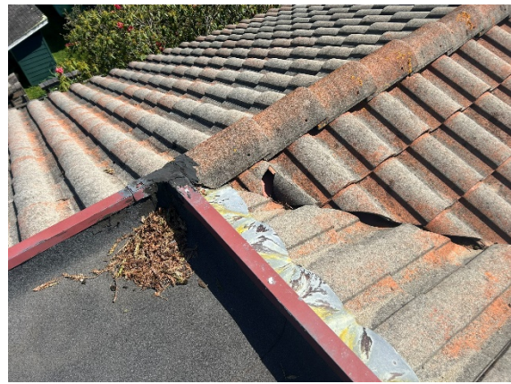
Figure 17 – Concrete S-Tile Roof
