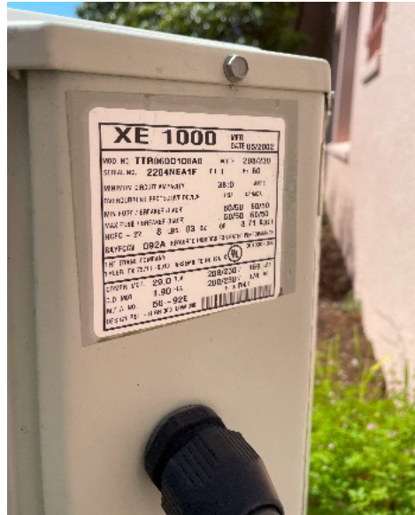
Figure 4 Condensing Unit Nameplate
