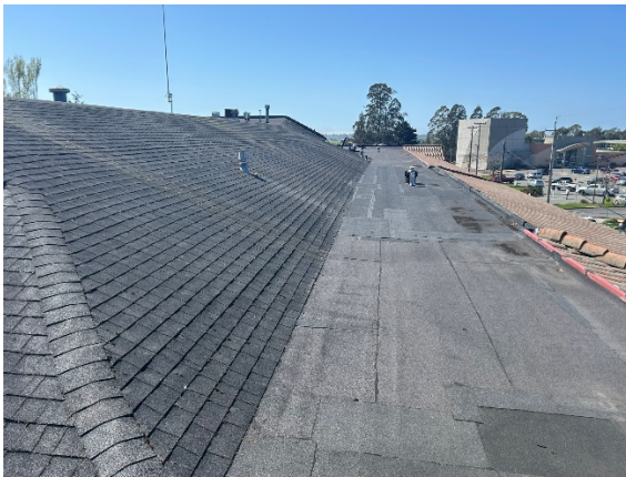
Figure 16 – BUR to Asphalt Shingle Roof Transition
