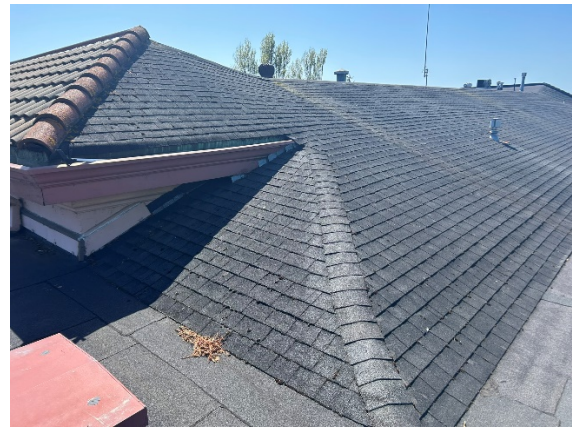
Figure 15 – Asphalt Shingle Roof at 'High Roof'
