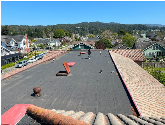
Figure 14 – BUR at Low-Sloped 'Low Roof'
