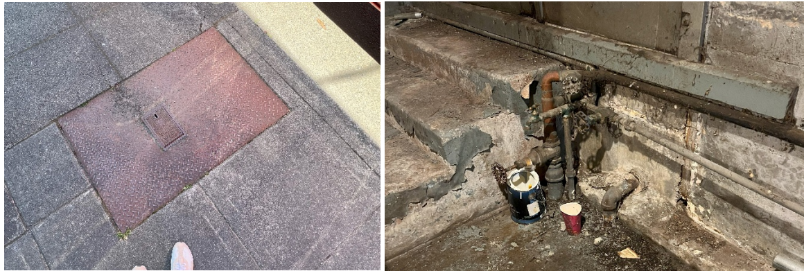
Above: Below-grade water meter and water service into building
