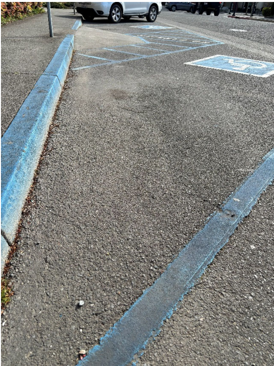
Photograph 6 – Rossow Street ADA stall – view looking south
