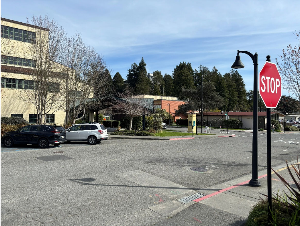
Photograph 7 – Rossow Street and SBS flatwork – red paint (typical) contains lead – view looking southeast
