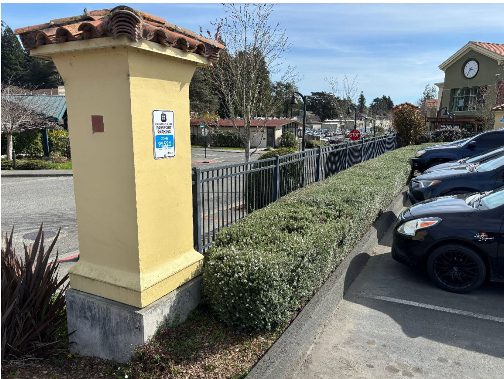
Photograph 8 – Parking Lot G11 retaining wall and curb – view looking southeast
